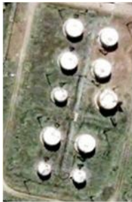
Figure 10. Storage tanks for petrol, oil and lubricants (POL)
